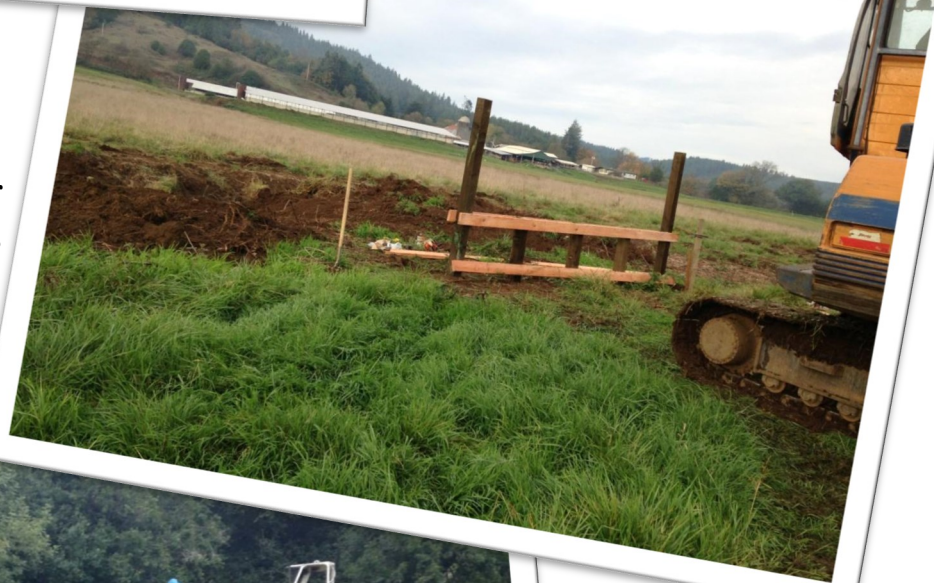
Project Implementation: construction of 'elk-braces' for wildlife stream crossings, Fall, 2016
