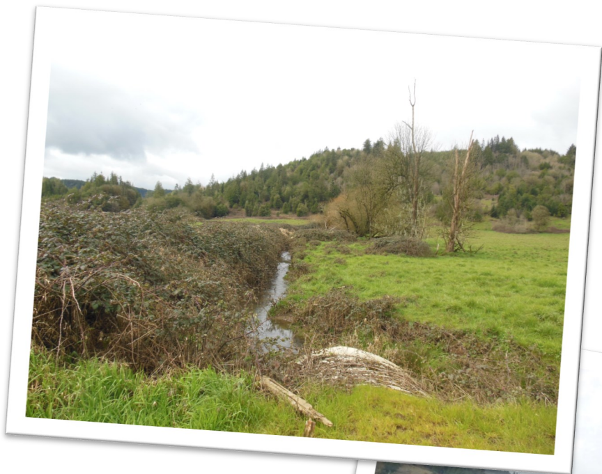
Wood Creek Pre-Project: degraded riparian, lots of blackberry, Summer, 2015
