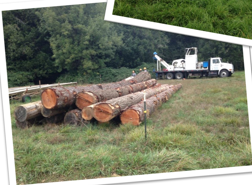
Project Implementation: logs piled and ready for instream placement, Fall 2015
