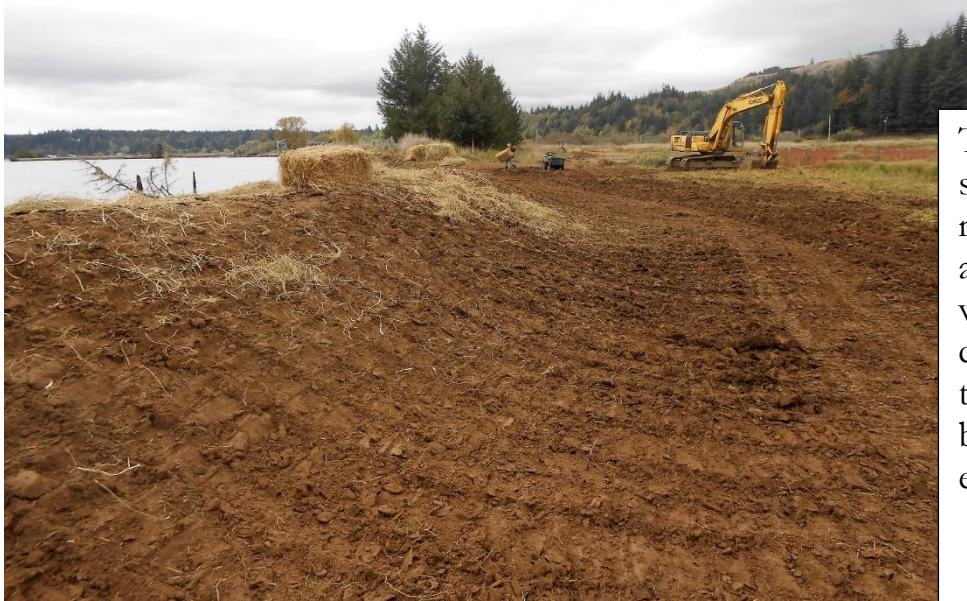
Last scoop of dirt from excavator seals the new and old dike.
