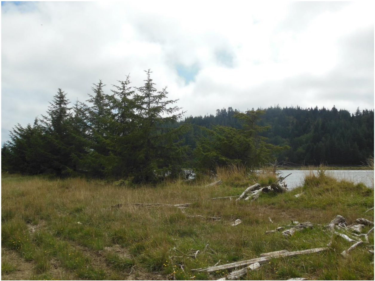
6. Section of existing diked river bank; note approx. 25 year old spruce trees toppling over due to being planted originally too close to the river and on top of the dike.
