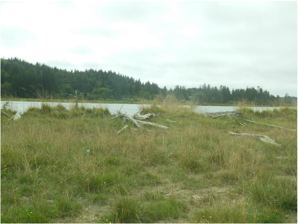
7. Failing section of dike photographed during summer months, 2014
