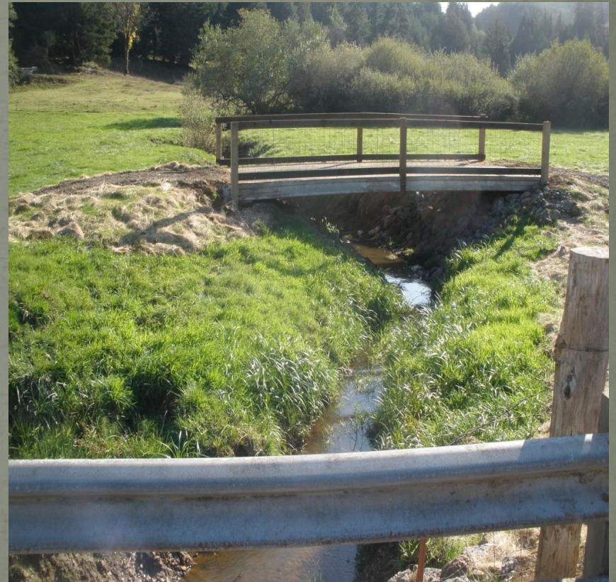
Standing on new bridge
