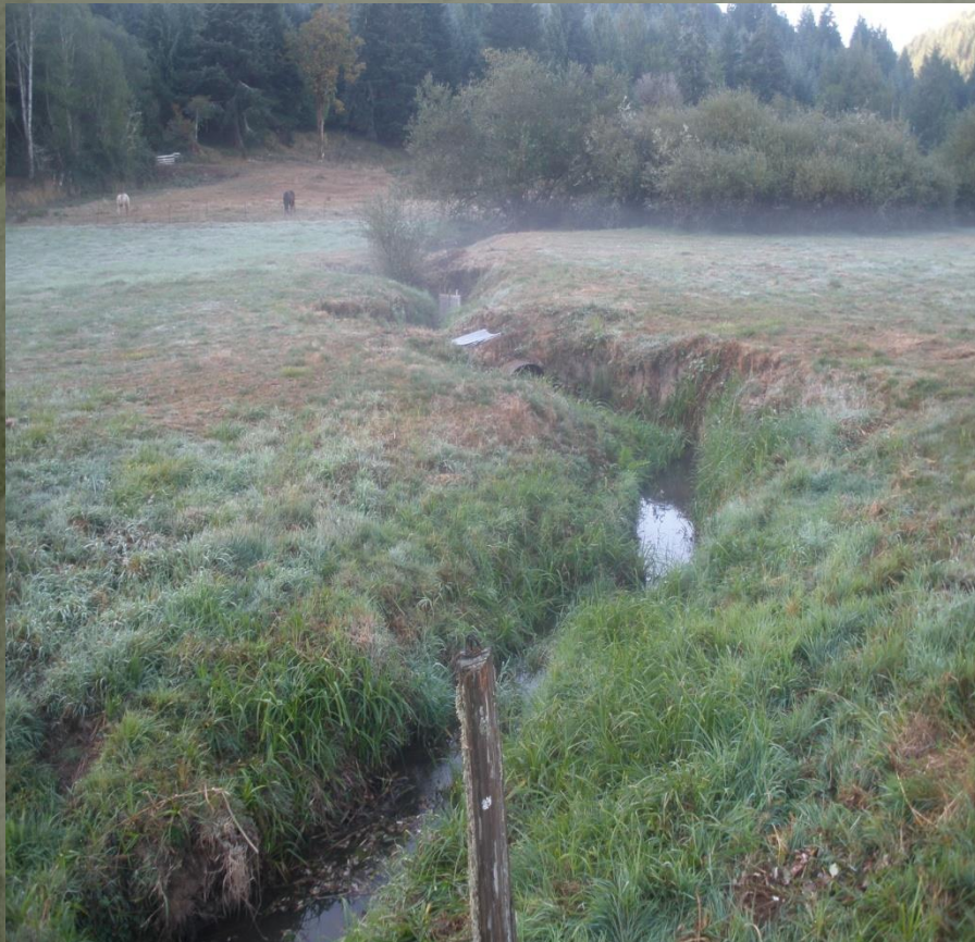
Standing on old culvert
