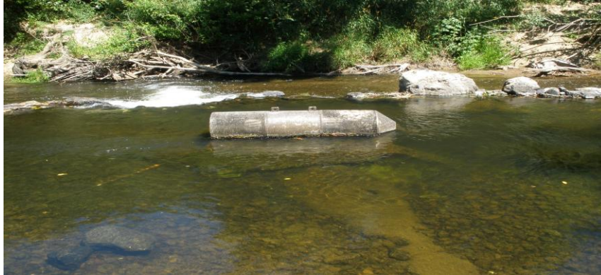
Myrtle Point's drinking water intake point with fish screen located on the North Fork of the Coquille River a 1/2 mile up Weekly Creek Road and the Cooper Bridge.
