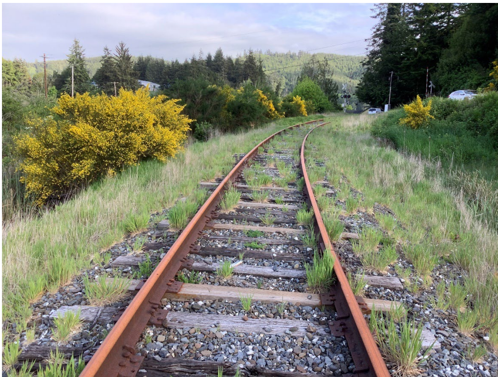
Overview of site 23-0250-01 north of the crossing, facing southeast.
