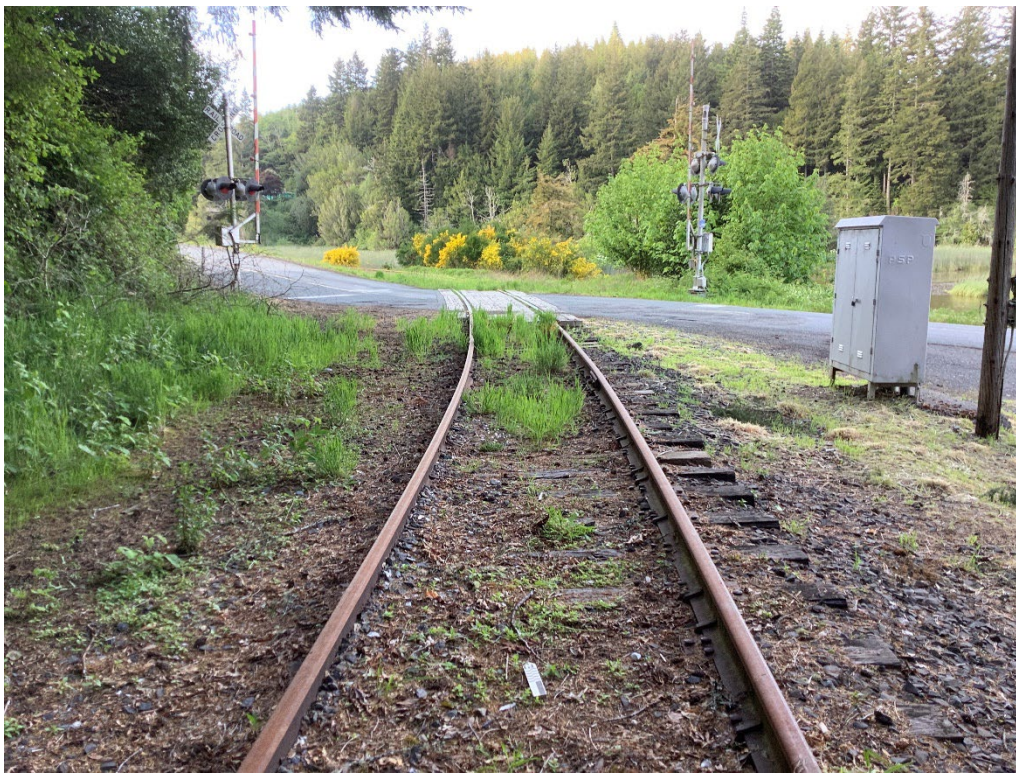
Figure 7-7. Overview of site 23-0250-01 from crossing, facing north
