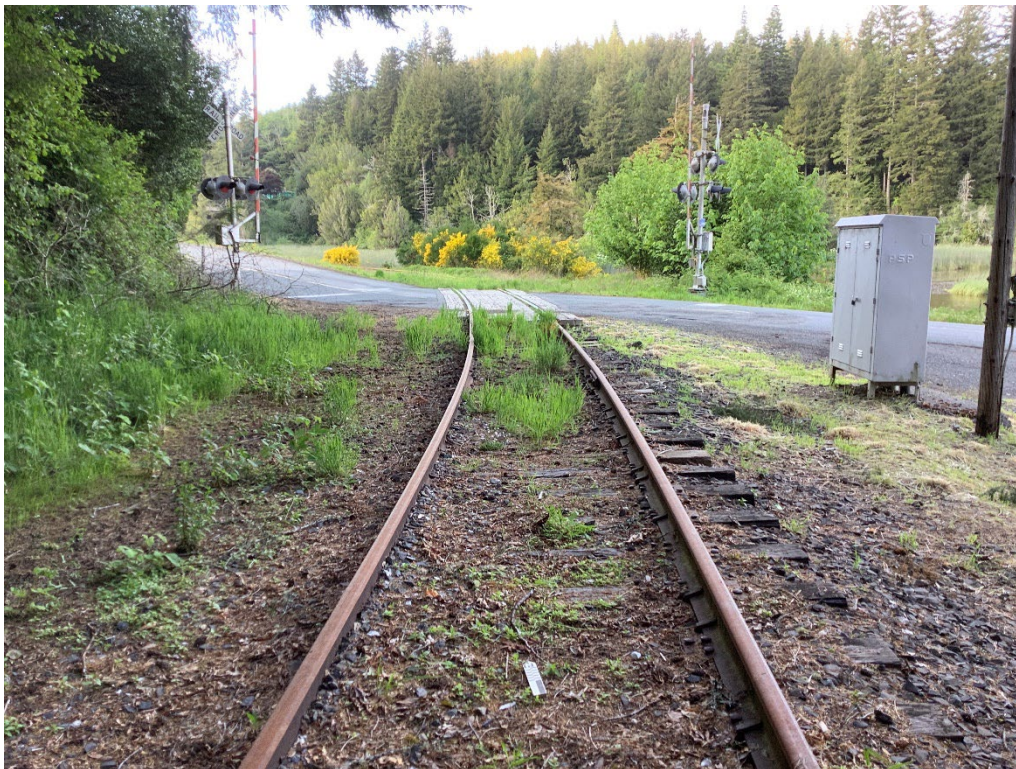
Overview of site 23-0250-01 from crossing, facing north.
