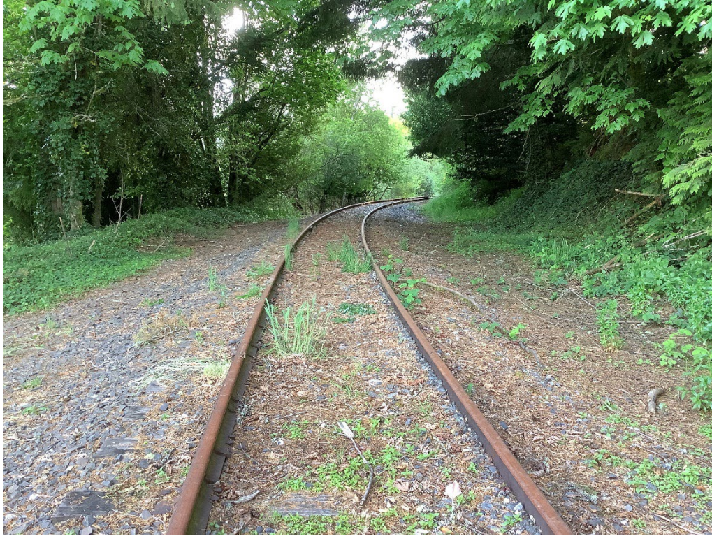
Figure 7-8. Overview of site 23-0250-01 from crossing, facing south.
