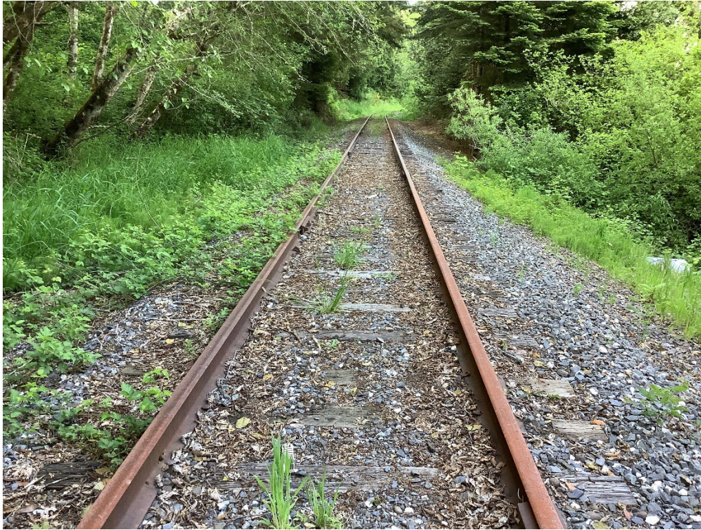
Overview of site 23-0250-01 from southern end in the APE, facing north.
