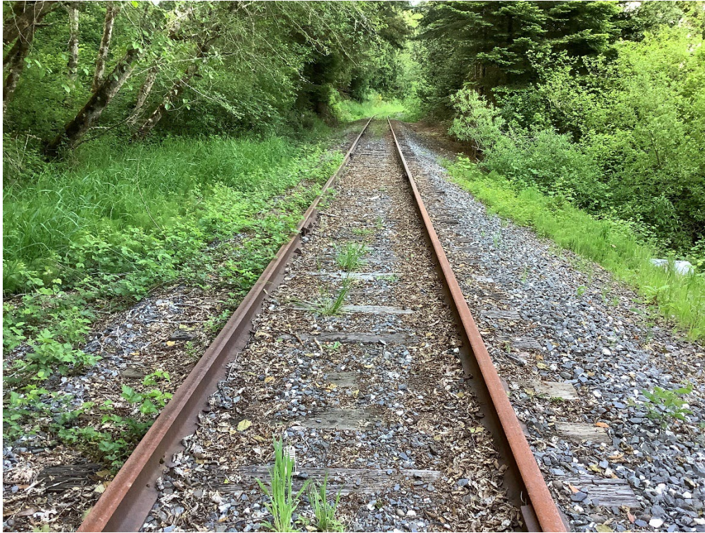
Figure 7-6. Overview of site 23-0250-01 from southern end in the APE, facing north.
