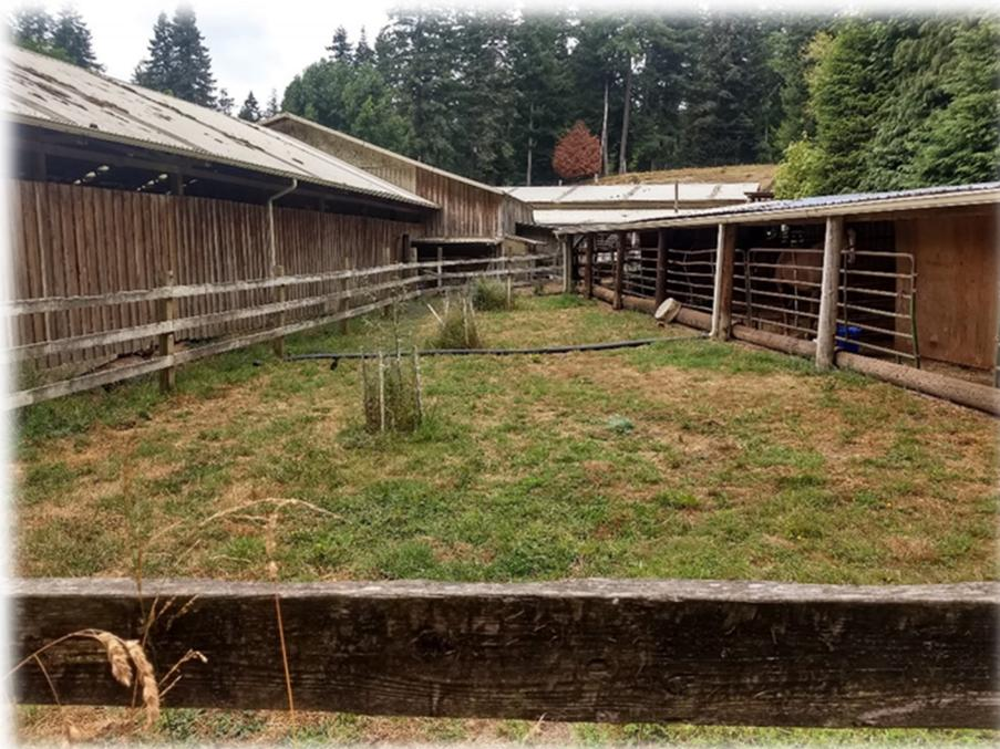
**Figure 16. (left)** Paddocks between barn and stables 2 years later: Roofing on paddocks still functional, vegetation is now established in between barn and paddocks. Gutters on paddocks are funneling water to the drainage area. (8/05/2020)
