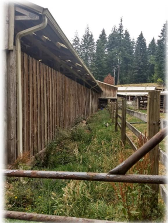
**Figure 19. (left) 2 Years later:** Main Barn gutters and adjacent drainage, vegetation has established in the area and is serving as a filtration system. (8/05/2020)
