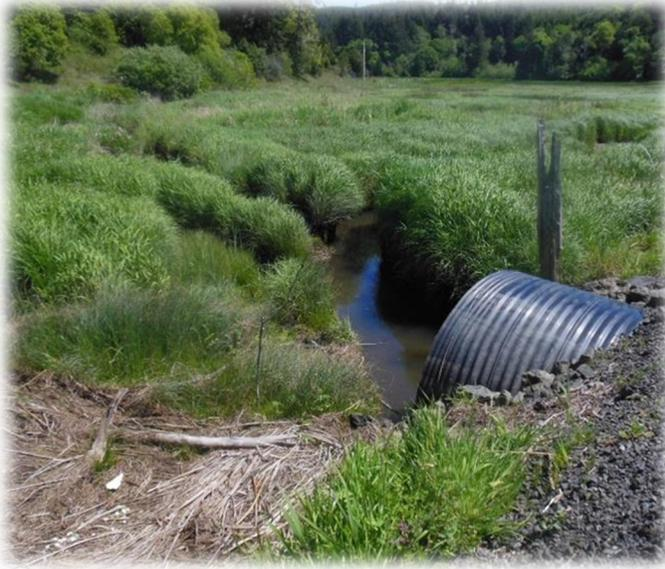
**Figure 6. (left)** This project was the site of a tide gate removal and culvert upgrade initiated by the County Road Department in 2016-17. Since installation of a larger pipe, the channel has begun flushing sediments and carving a more defined network in the lower portion of the pasture. This photo shows the new culvert and salt marsh tidal habitat post-fencing. (05/2018)
