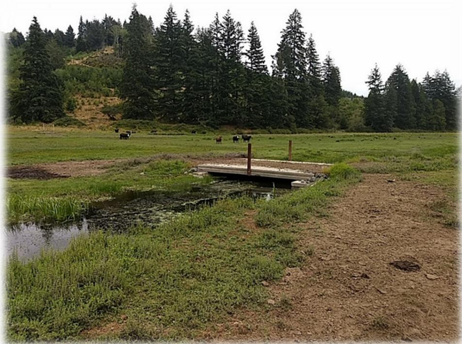
**Figure 35.** Two years after bridge implementation, crossing is still in good standing and the channel is becoming more defined. (8/05/2020)
