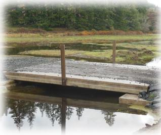
*Collapsing culvert replaced with concrete slab bridge at a livestock crossing.*
