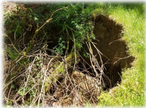
Forest Access road erosion due to collapsed culvert- Pipe Outlet (5/09/2019)
