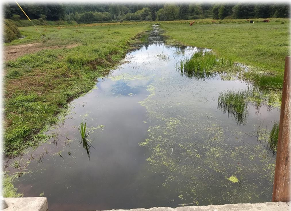
**Figure 33.** Adams Creek Main Channel inlet, 2 years after bridge installation (8/25/2020). Water levels may be higher this year, however the channel has clearly flushed some of the sediments and there is less vegetation in the channel. This indicates improved movement and sediment exportation.
