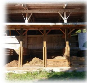
*Four-bay manure storage and composting facility installed at a local horse boarding operation*
