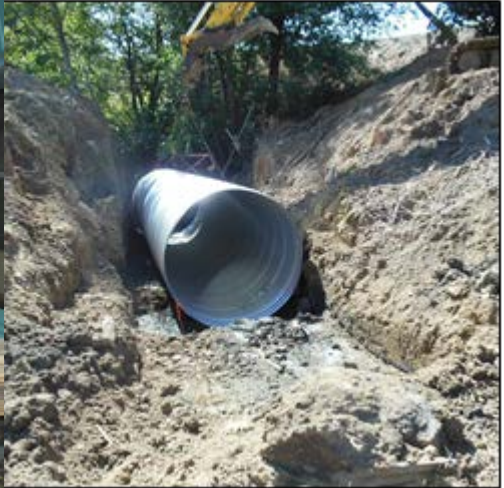
The photos above show the new culvert being put into place.
