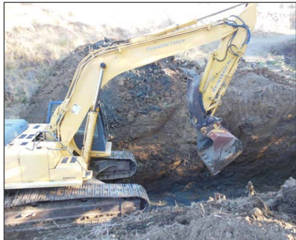
The above photos show the wreckage of the school bus after it was removed in pieces, and an excavator digging out the trench for the new culvert to be placed in.
